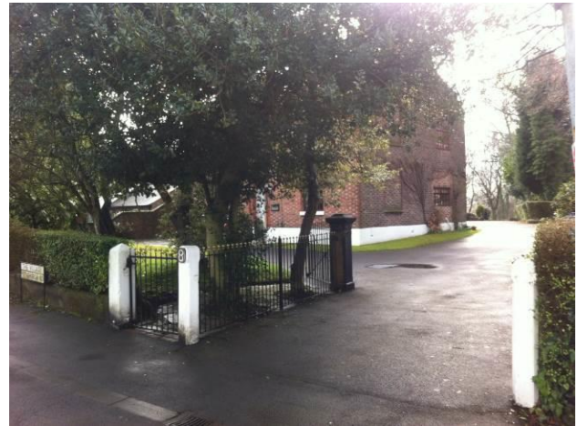
Inappropriate railings and historic gate piers at Holly Bank
