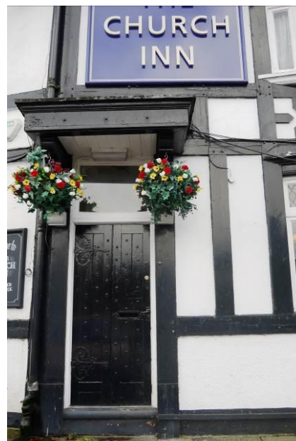
Traditional vernacular features on The Church Inn
