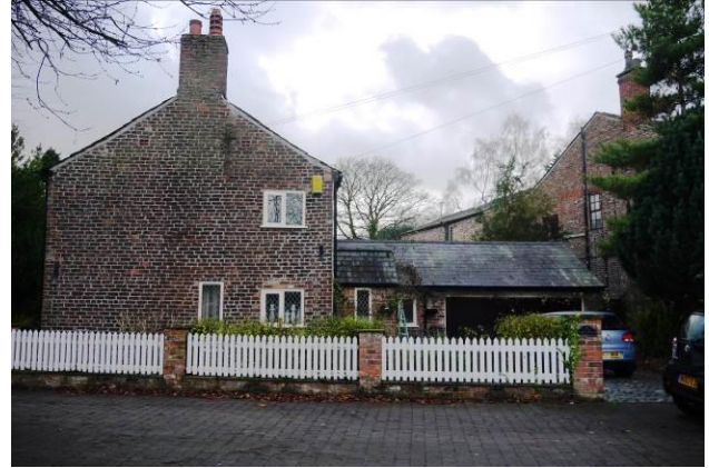
Use of local brown brick as a prominent building material at no. 16 The Village
