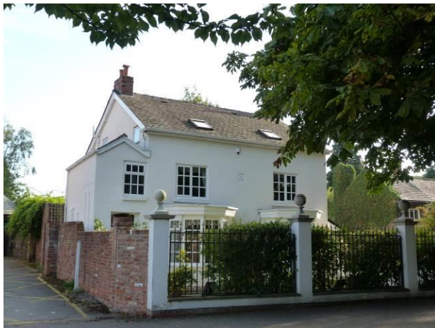
Inappropriate boundary treatments at 22 The Village
